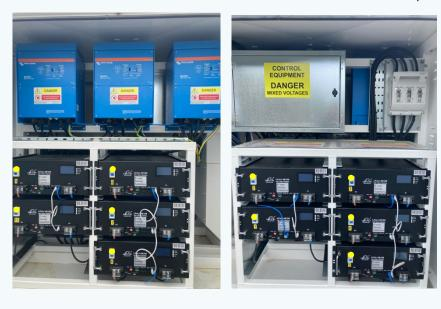
4 – Hold down the 'reset' buttons on all 10x batteries until the lights switch OFF. (marked in red dots below). (Batteries found on both sides of the pod)
