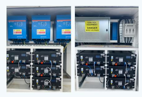
5 – Once ALL batteries fully switched off the pod is ready to be towed.
