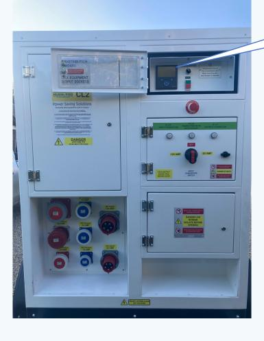
6 – Switch the 3x inverters (blue boxes) to the 'ON' position starting with the left hand one and work right. (N.B. They never need to be on the 'charger only' position)
